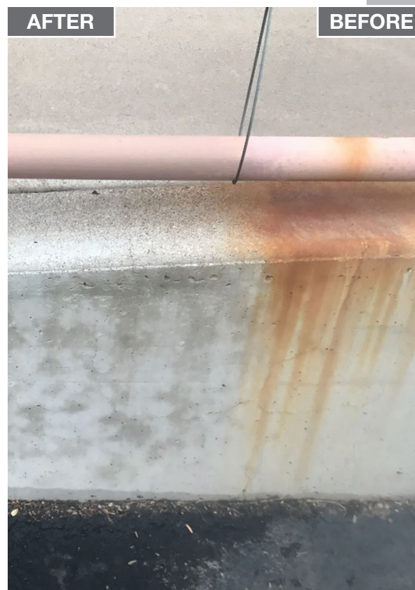
BARC Process #2 on Concrete Mighty Mobile Power Wash Lake Havasu, AZ
