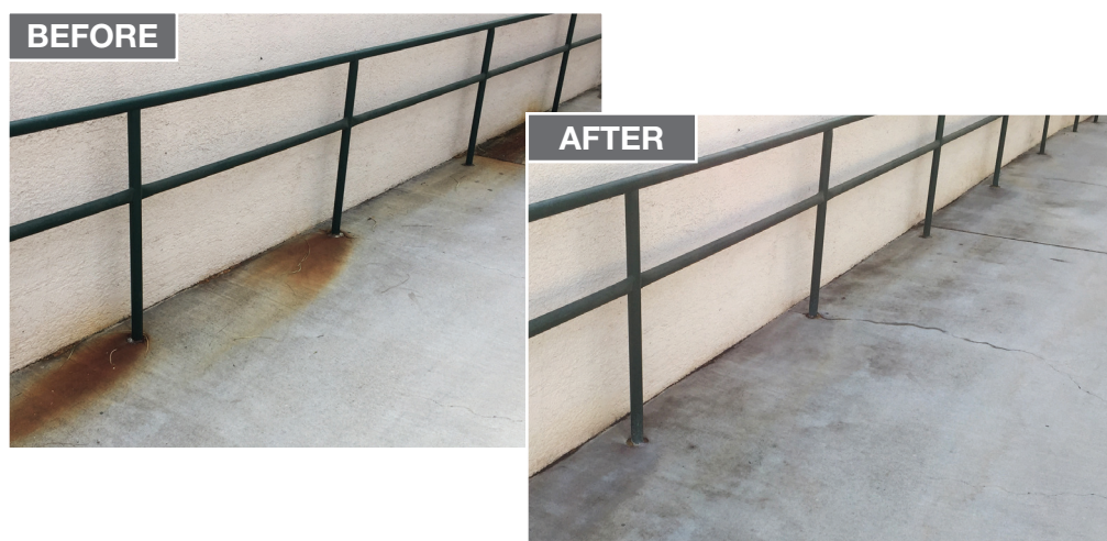
BARC Process #1 Rust from Metals Innovative Cleaning Services Phoenix, AZ
