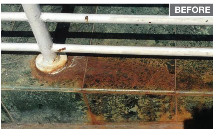
BARC Process #1 Heavy Rust on Granite
