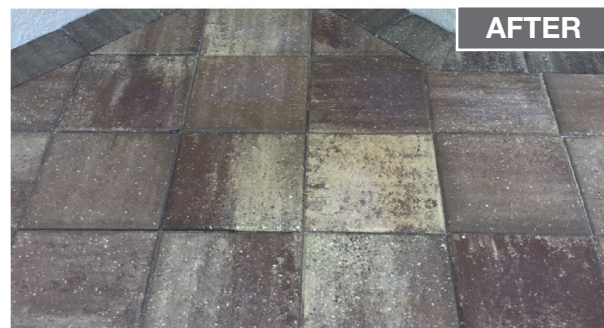
BARC Process #1 Heavy Rust and Fertilizer Rust Stains Spray Soft Exterior Cleaning Smyrna Beach, FL
