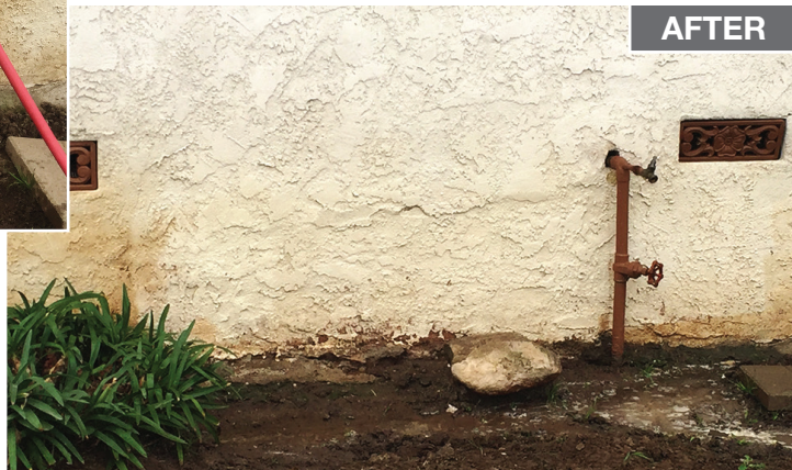
Efflo Process #3 Mud Stain on Stucco A3 High Pressure Cleaning Carson, CA
