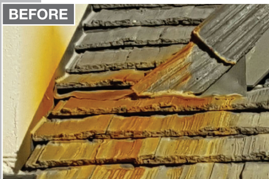
Rust on Asphalt Roof Shingle Cajun Soft Wash Baton Rouge, LA
