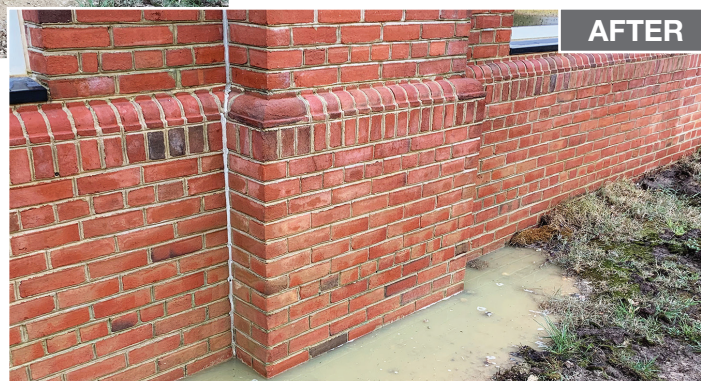
F9 Efflo Process #3 On Point Exterior Services St. Mary's County, MD
