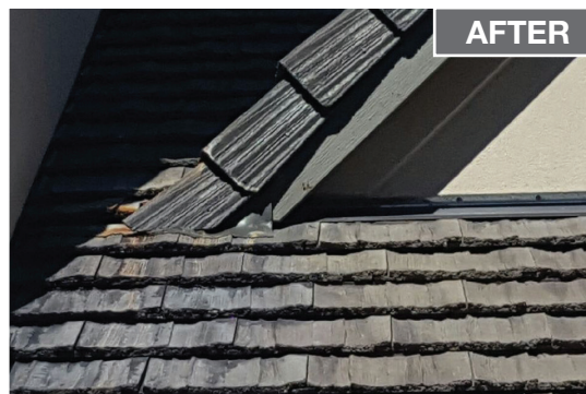
Rust on Cedar Shake Shingle
