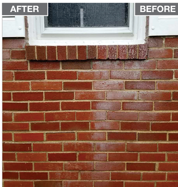
BARC Process #3 for Window Frame Paint Oxidation Runs The Roof Wizard, LLC Hammonton, NJ
